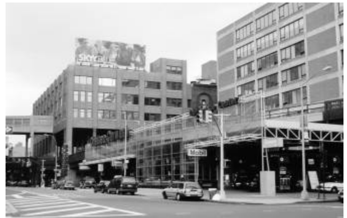
Fig. 5. Scaffold (performing as carwash) applied to Highline
