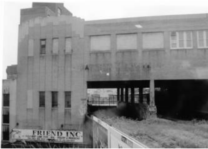
Fig. 7. Building void along Highline, Manhattan
