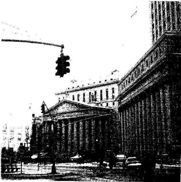
Fig. 9. View from Foley Square towards New York County Courthouse and the United States Courthouse.
