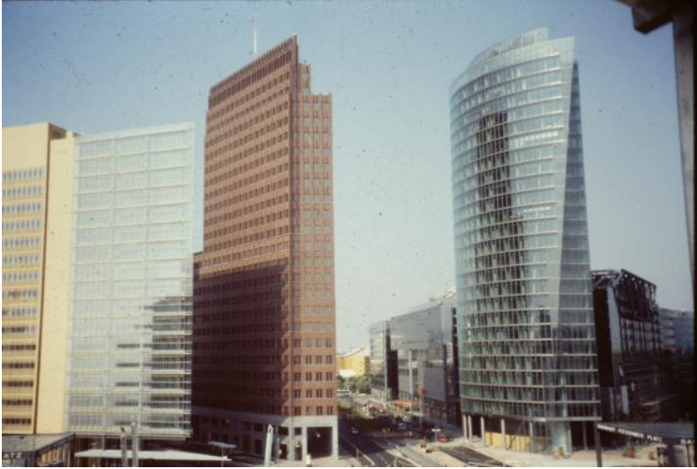
Towers by Murphy/Jahn on right, Hans Kollhoff on left
